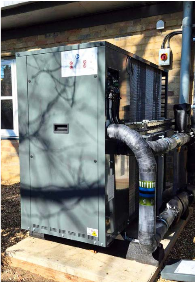
ATEX zoning requirements are displayed on all heat pumps featuring R290 natural refrigerant.
