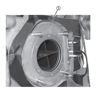
With the burner removed the heat exchanger may now be cleaned. To remove any debris flush the heat exchanger with water, if possible from a pressurised supply, taking care to protect any electrical components against moisture. Ensure the heat exchanger is fully flushed.
