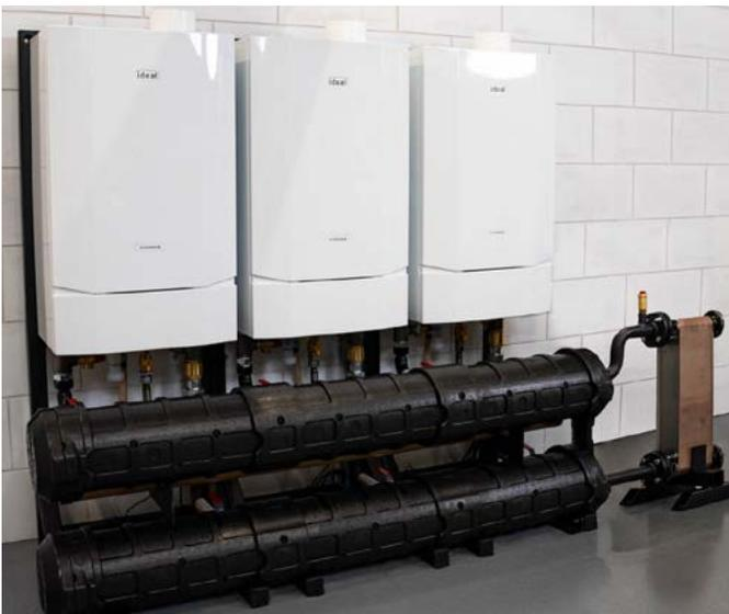
With a large single boiler, it would cycle on and off, using considerably more fuel than strictly necessary.
