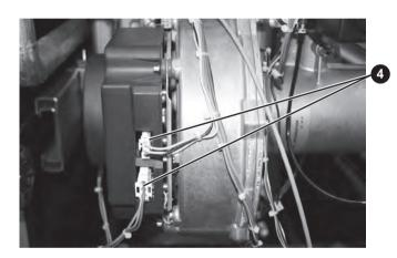
5. Disconnect the detector lead 'in line' connector.
