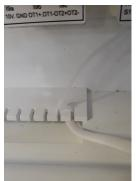
7. In the case of a Slave boiler, route the CANBus RJ11 cable into the bulkhead and connect and secure as above.
